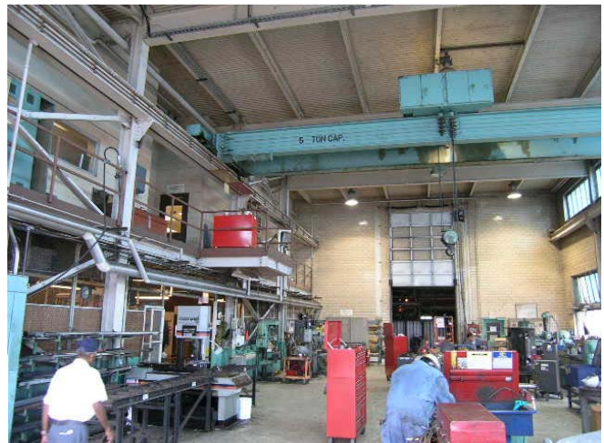
One bay was added to the maintenance shop.
